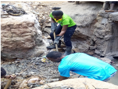
Students unblocking a drainage channel
