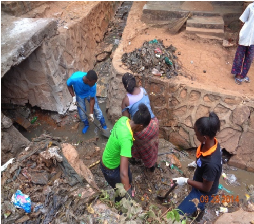
Environmental health students unblocking one of the drainage channels
